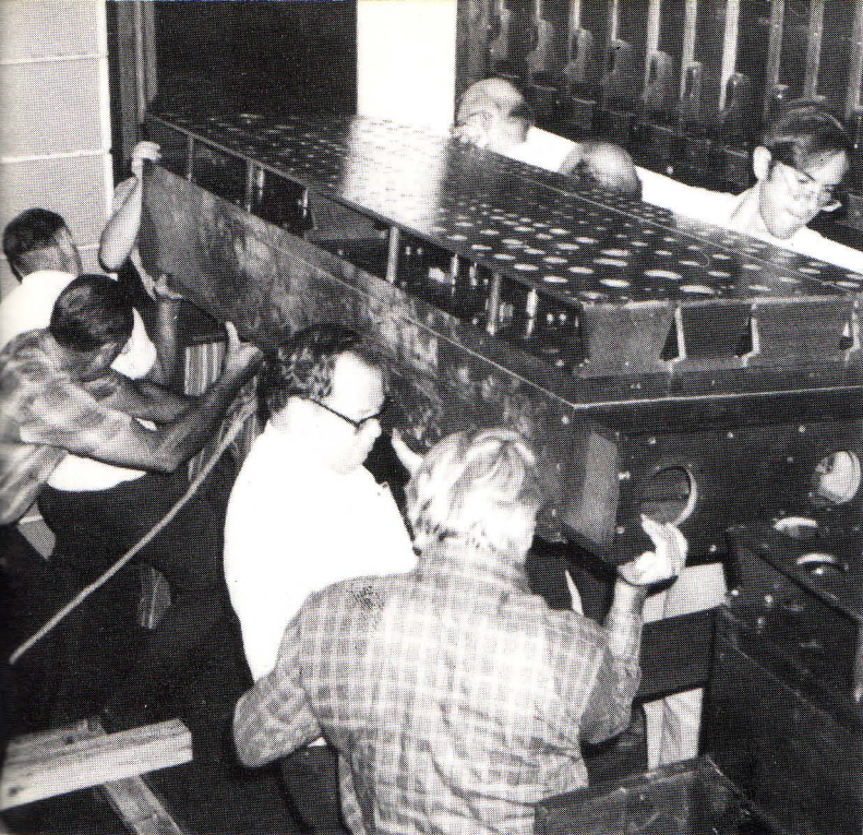
Easing a four rank chest into place in the Main Chamber.
