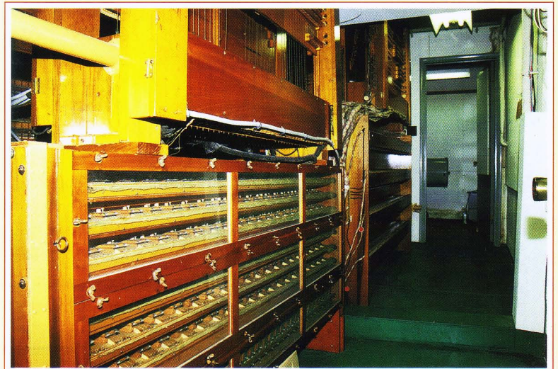
Relay room—blower room in back.
